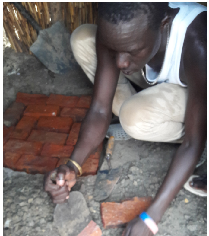
Rubkona Rocket stove construction in the shade in the PoC site. A total of four stoves were constructed.
